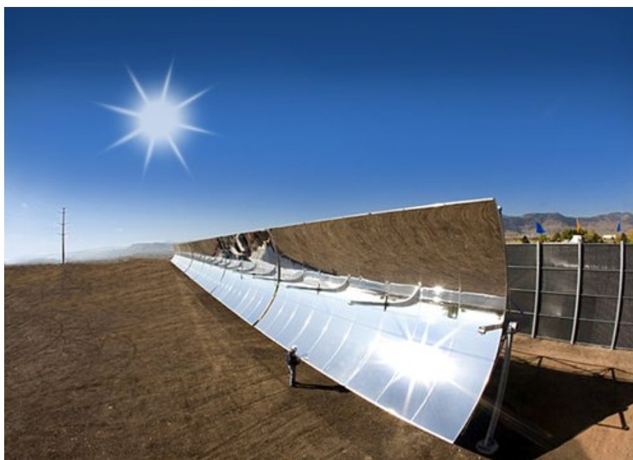
Figure A-4. SkyFuels' SkyTrough large-scale parabolic trough
