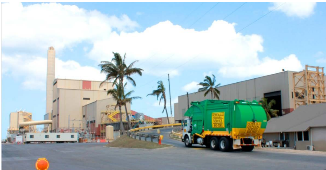
Figure 20. 50 MW waste-to-energy facility in Oahu, Hawaii
